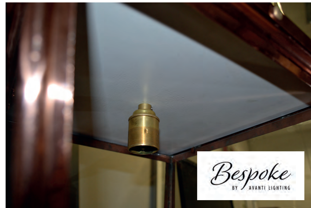
New internal baffle plate and lampholder installed.
