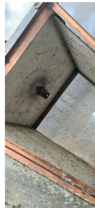
Old internal baffle plate and lampholder.
