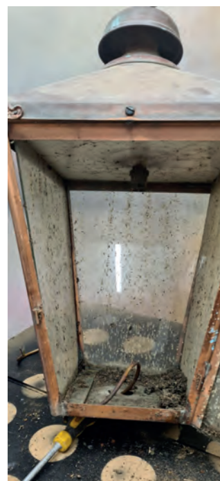
Cleaning out the insides and stripping out the old wiring.
